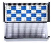
The subscriber connector block is used to terminate field monitoring device pairs on subscriber circuits. It routes incoming jumpers from the vertical frame to the subscriber card in the 289H/H-M monitor and to the central office equipment. Wire wrap termination pins are divided into two groups—each to accommodate 25 devices on subscriber circuits.
